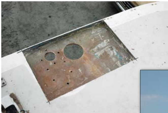
Old and new holes for davit compression post
