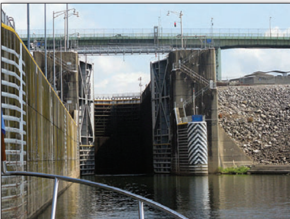
Ft. Loudon Lock
